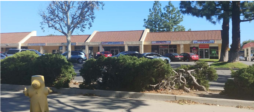
Typical retail building condition (Tapo Street Corridor): 1-story building with multiple tenant spaces separated from the sidewalk by surface parking
