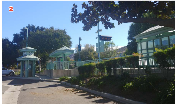
Metrolink Station Source: Gruen Associates
