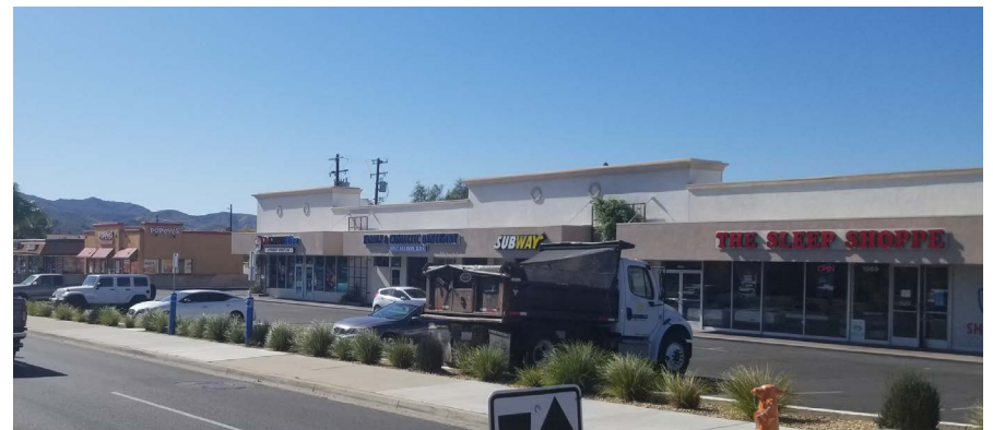
Typical retail building condition (Los Angeles Avenue Corridor): 1-story building with multiple tenant spaces separated from the sidewalk by surface parking
