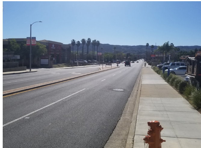
Erringer Road is a four-lane secondary arterial with a turn lane and median
