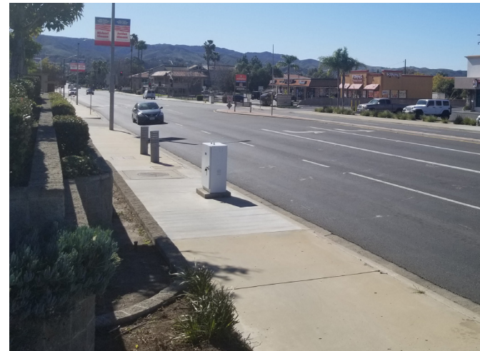
Narrow sidewalks along Los Angeles Avenue with buildings that don't address the street
