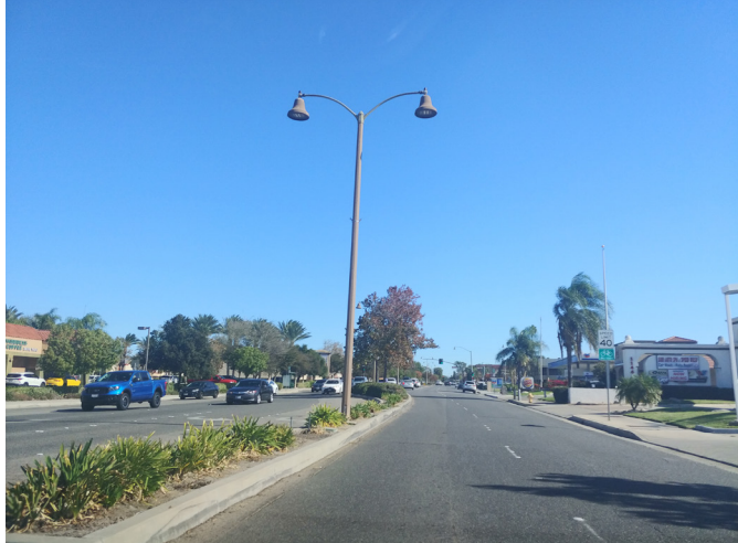
Los Angeles Avenue is a six-lane primary arterial with a landscaped median, relatively narrow sidewalks, and bike lanes that don't extend into our boundary
