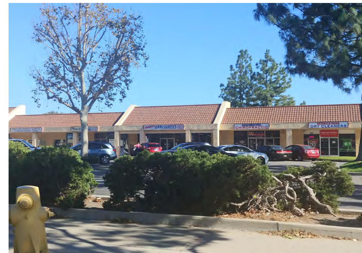
Typical retail building condition: 1-story building with multiple tenant spaces separated from the sidewalk by surface parking
