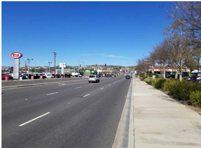
First Street is a six-lane primary arterial with a turn lane and median north of Los Angeles Avenue and transitions to a four-lanes south of that intersection
