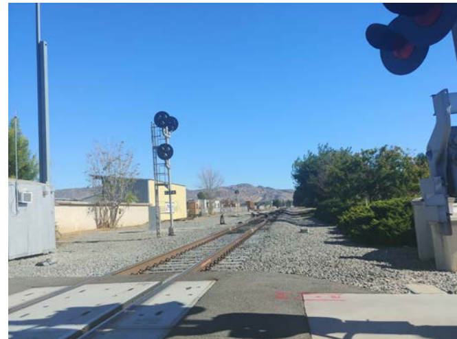
Metrolink rail right-of-way
