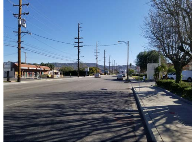
Cochran Street is a four-lane secondary arterial with no median or bike lanes
