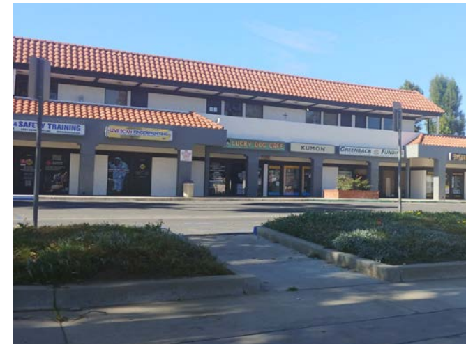
2-story retail building in Tapo Street Corridor
