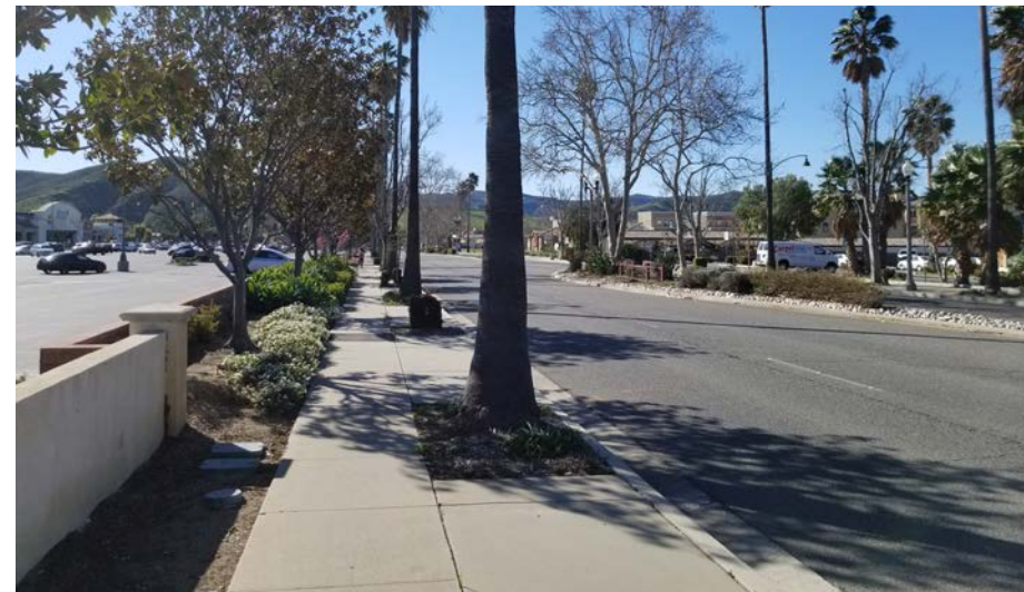
What Tapo Street (between Cochran and Alpine) looks like today
