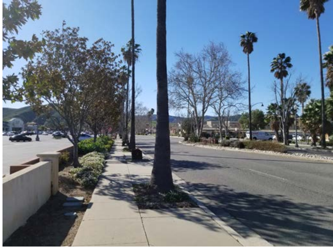
Tapo Street is a four-lane secondary arterial with a landscaped median and reduced speed limits between Los Angeles Avenue and Cochran Street
